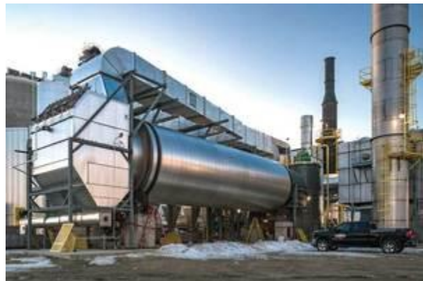
Thompson Dryers, which has been in industrial drying for 75 years, is installing its Thompson Phytosanitary System at New England Woodchip Solutions LLC, collocated at the site of Orrington, Maine-based Penobscot Energy Recovery Co.
